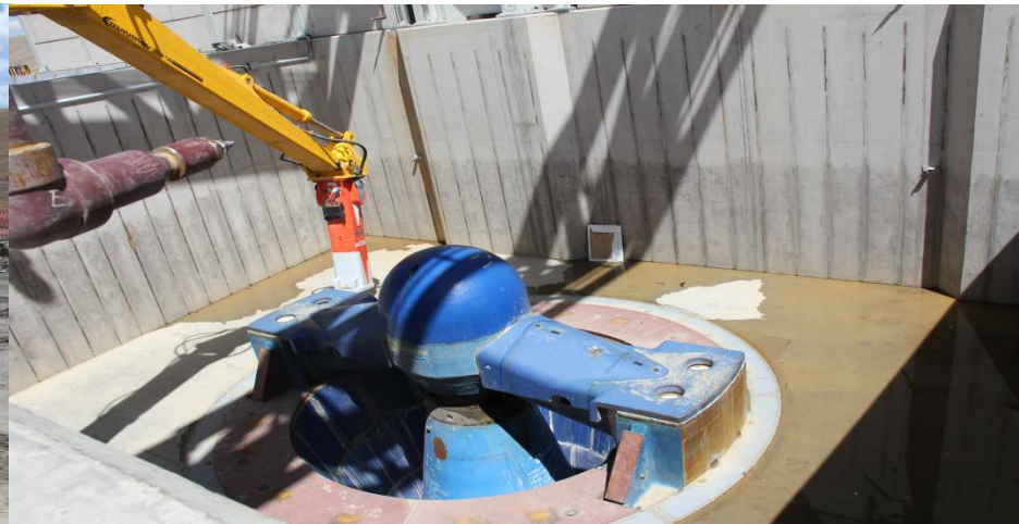
Constancia ore dump pocket for the primary crusher
