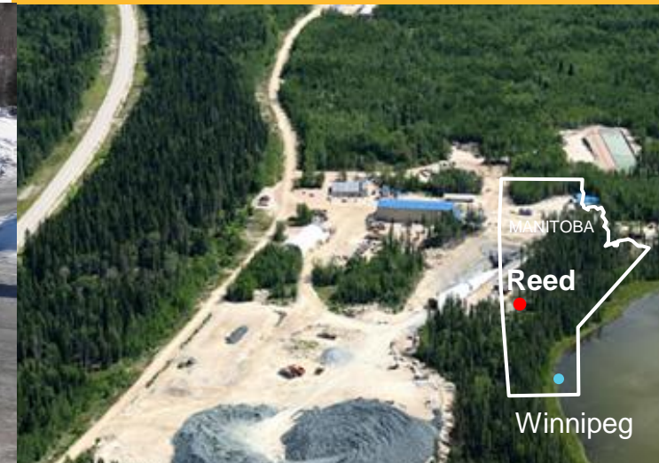
Aerial view of Reed project site
