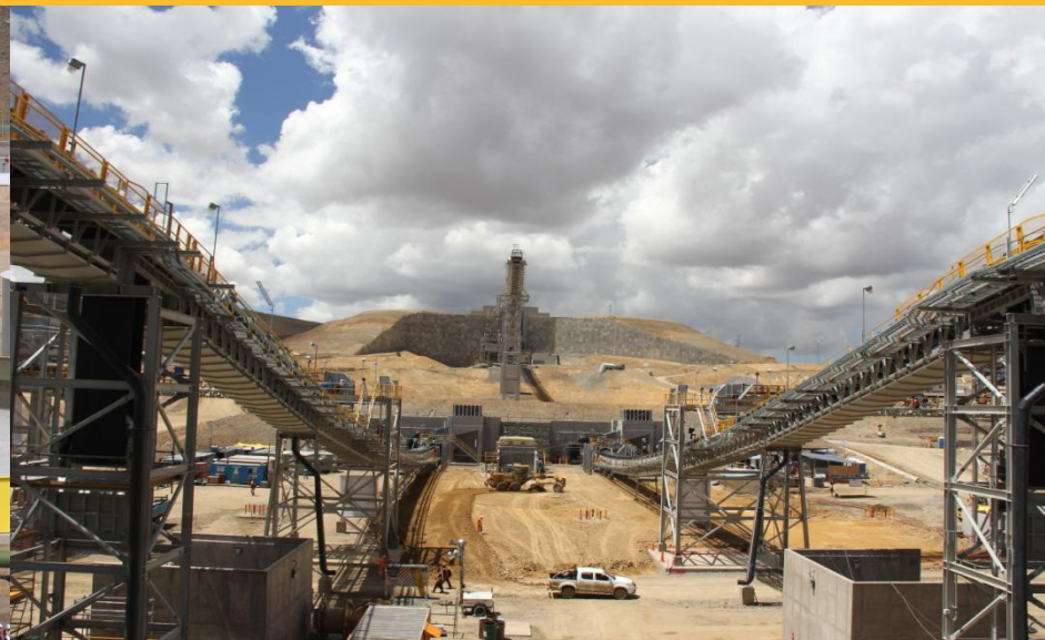
Crushed ore stockpile reclaim tunnels to feed ball mills
