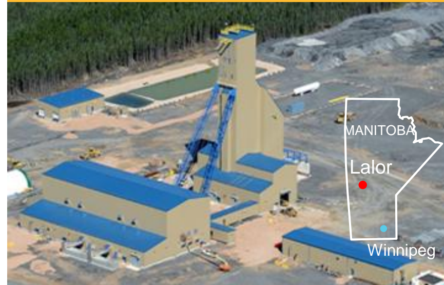
Aerial view of Lalor project site
