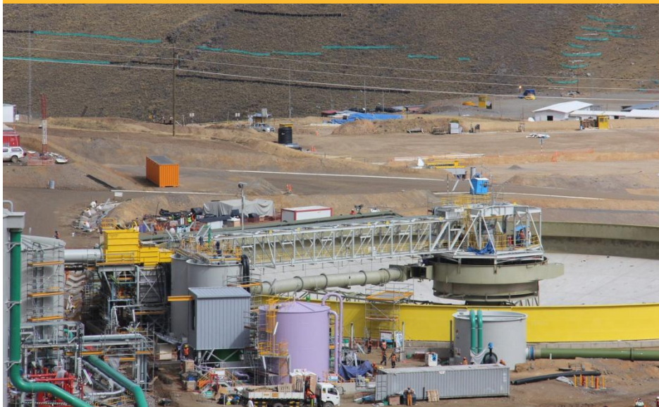
Constancia tailings thickener
