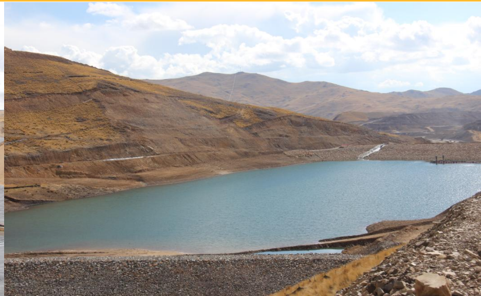
Constancia main sediment pond
