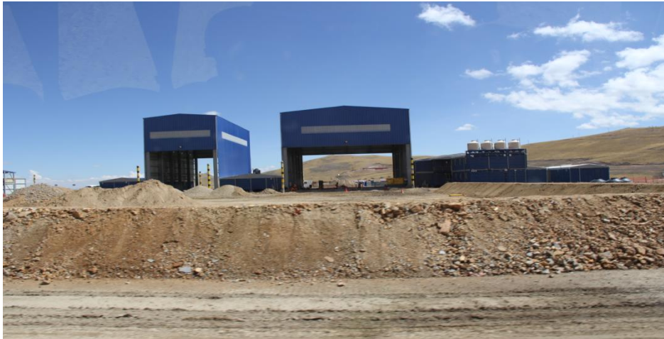
Constancia mine maintenance facilities
