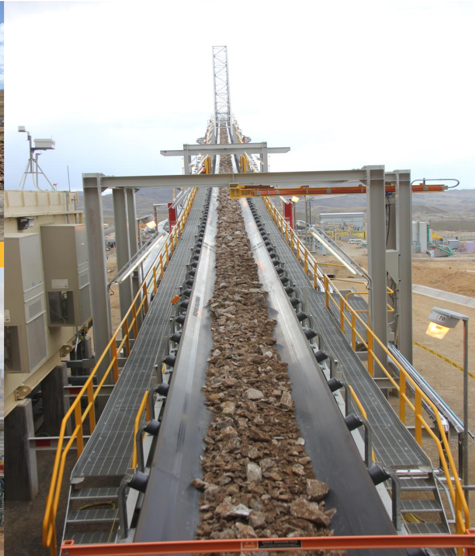
Commissioning of Constancia crusher
