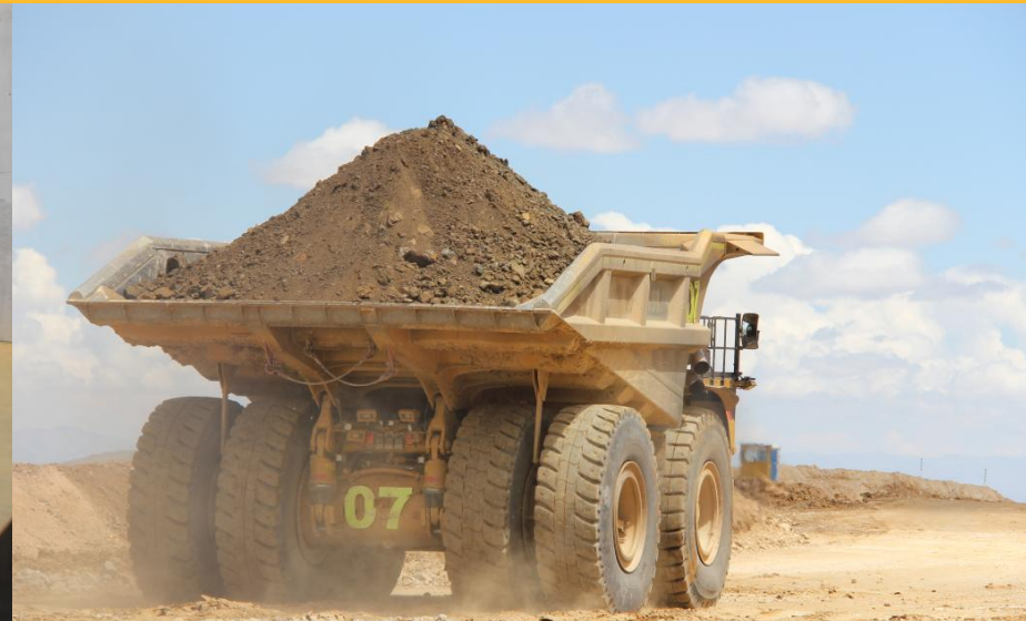
Pre-stripping activities at Constancia
