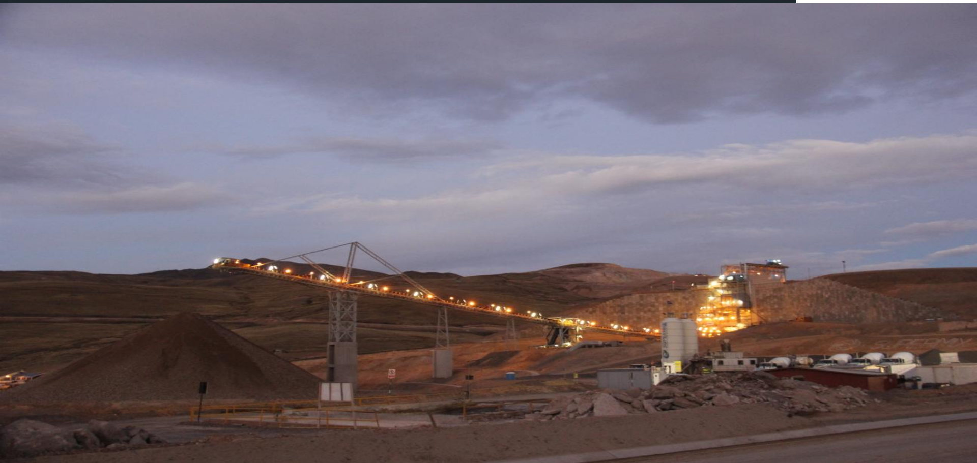
Night view of Constancia crusher
