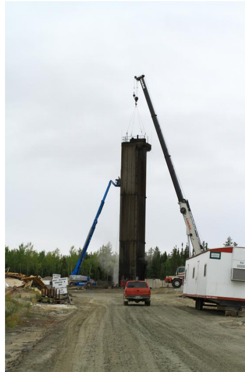
Demobilization of temporary hoist
