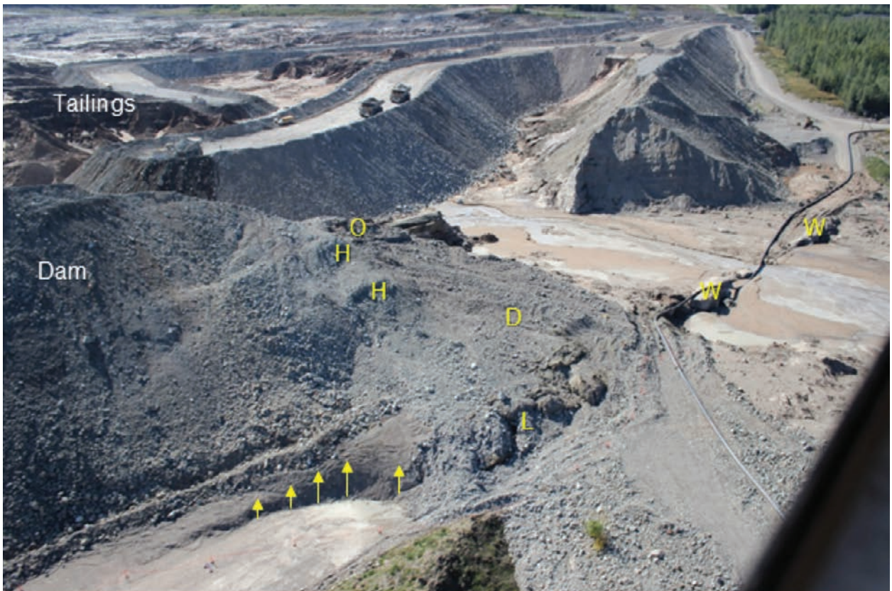
FIGURE 5.1.6: SLIDING-RELATED FEATURES AT RIGHT ABUTMENT (SEPT. 4, 2014 PHOTO)
