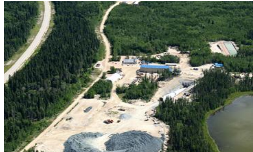
Aerial view of Reed project site
