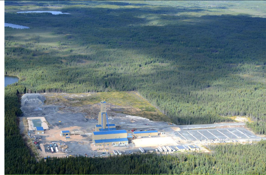
Aerial view of Lalor project site
